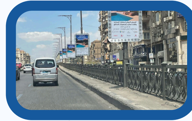
NOZHA BRIDGE Heliopolis
